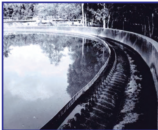
Fig 13.5 : Water clarifier
